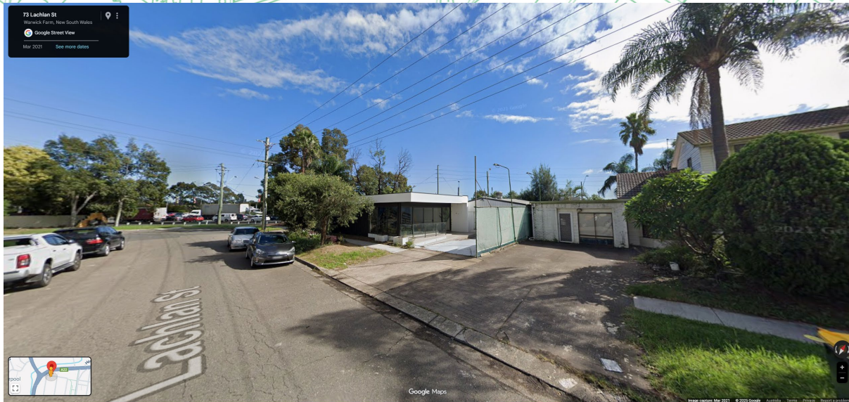
Figure 6. Google Street View image of the Site and streetscape from Lachlan Street (Extracted from https://www.google.com/maps/place )
